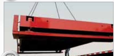
2 Unload and set modules.
