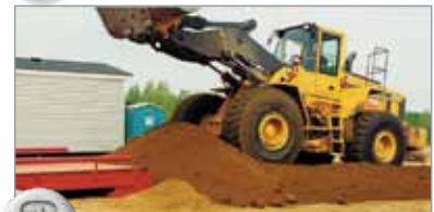
3 Backfill to bulkheads and finish ramps.
